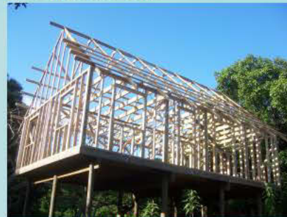
2010 Missions in Roatan, building a home.
